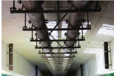
Pipeline running underneath a bridge.
