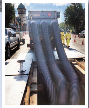
40,000 cf dust collectors from Rapid Prep are ideal for cleaning large diameter pipelines. They save time and are highly efficient.
